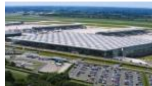
Stansted Airport Grade E
